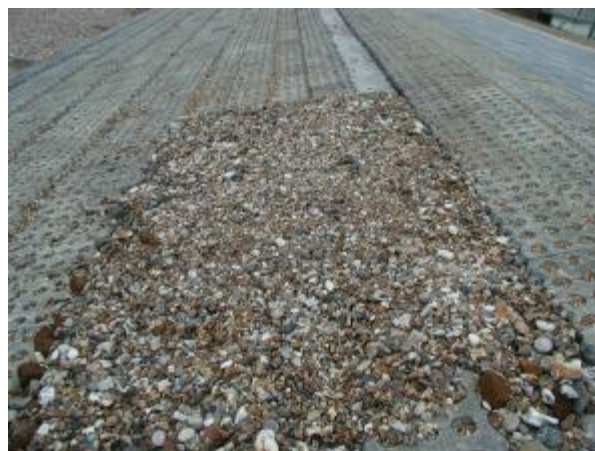
Figure 2: Small shingle patch on the Southern Revetment where the Oystercatcher nest is located
